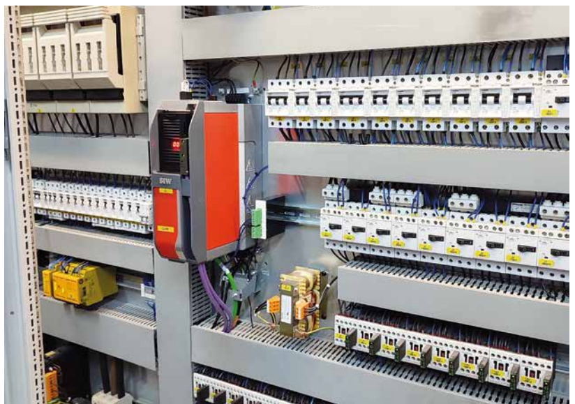
New inverters for conveyor drives
