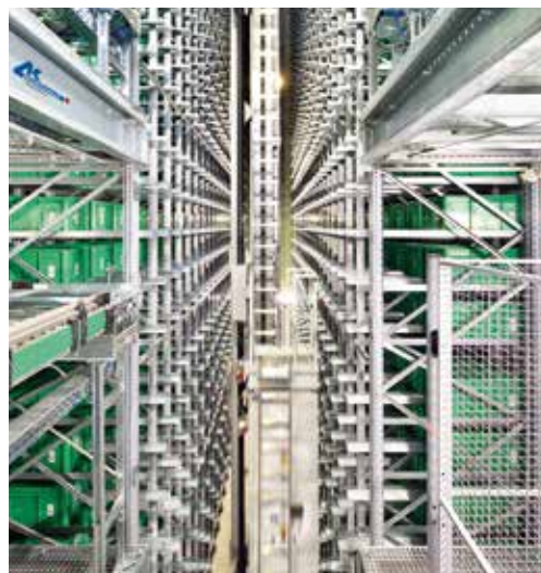
Automated small-parts warehouse for 8,800 containers
