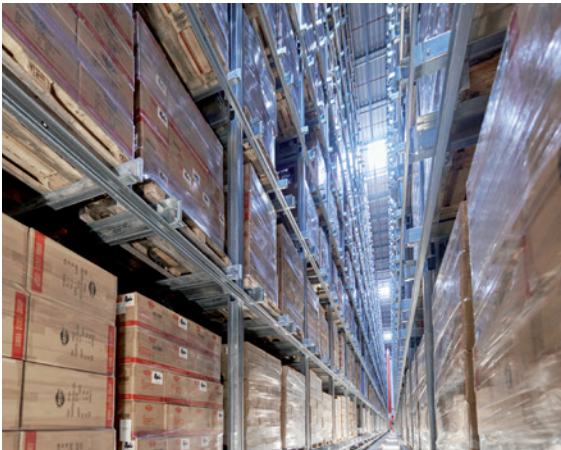
2-aisle, fivefold-deep channel storage
