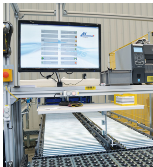
Order picking workstation with warehouse management system
